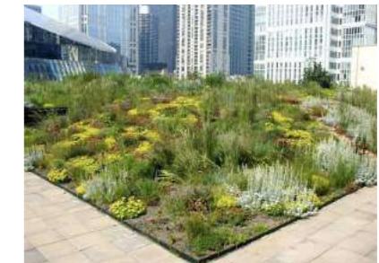
Figure 34: Green roof above Chicago's City Hall market.
