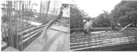
P.T. BEAM BEING LAID DOWN ON THE SECOND FLOOR SLAB
